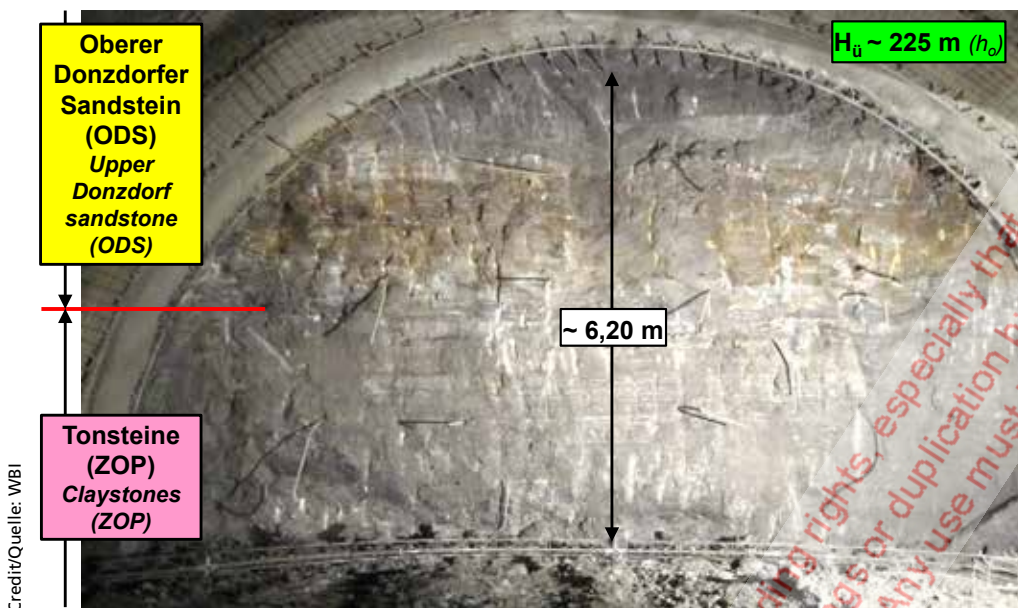
11 Eastern tube, photograph of the temporary face at tunnel meter 709.4
