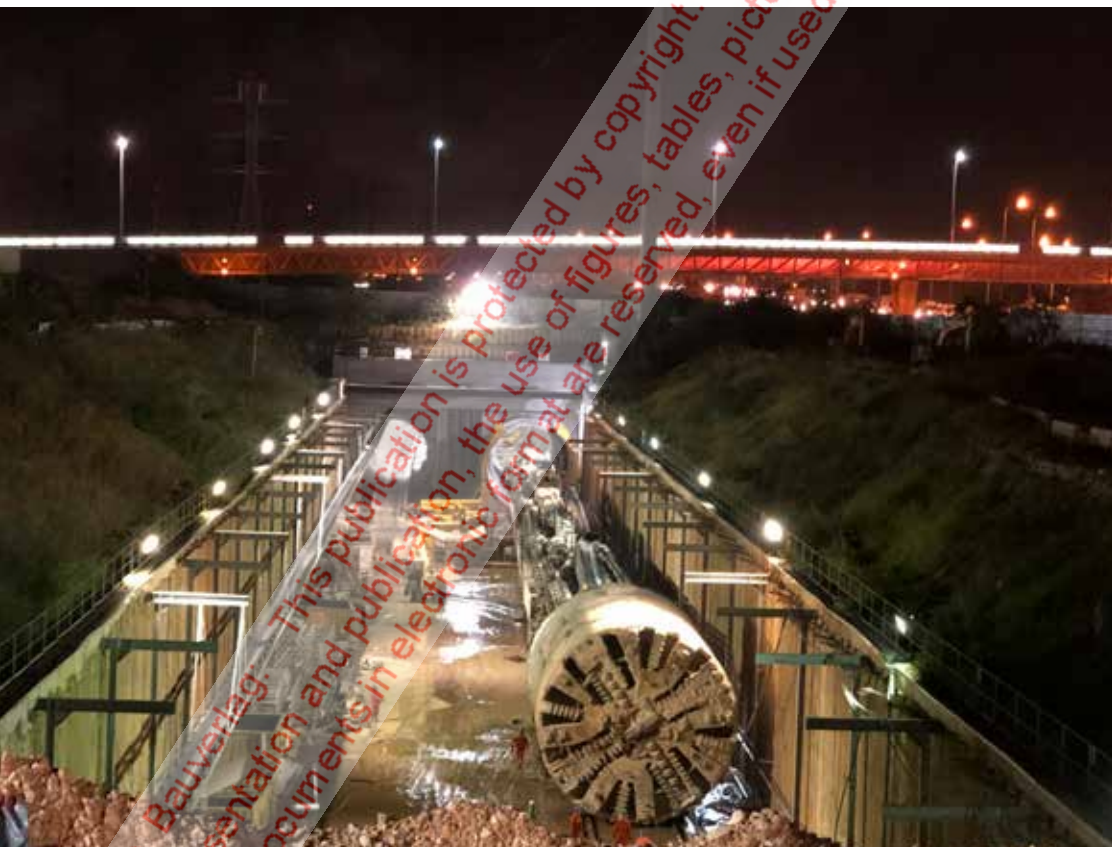
5 TBM S1027 inside Em Hamoshavot Station (left) and view into tunnel at Depot Portal (right) TBM S1027 in der Station Em Hamoshavot (links) und Blick in den Tunnel am Depot-Portal (rechts)
