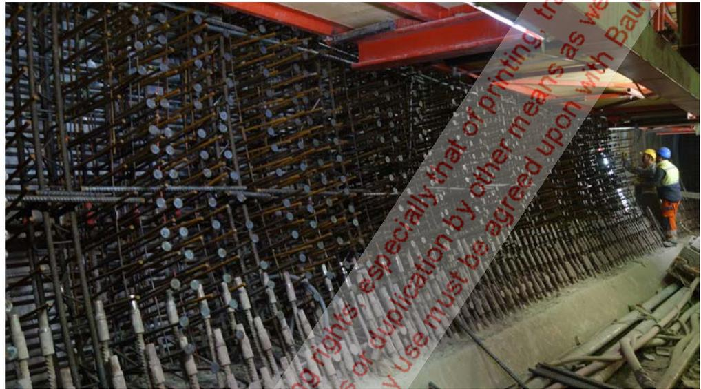
12 Reinforcement in the sidewall, example Feuerbach Tunnel
