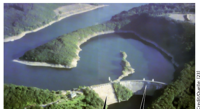
25 Urft dam and reservoir Urfttalsperre
